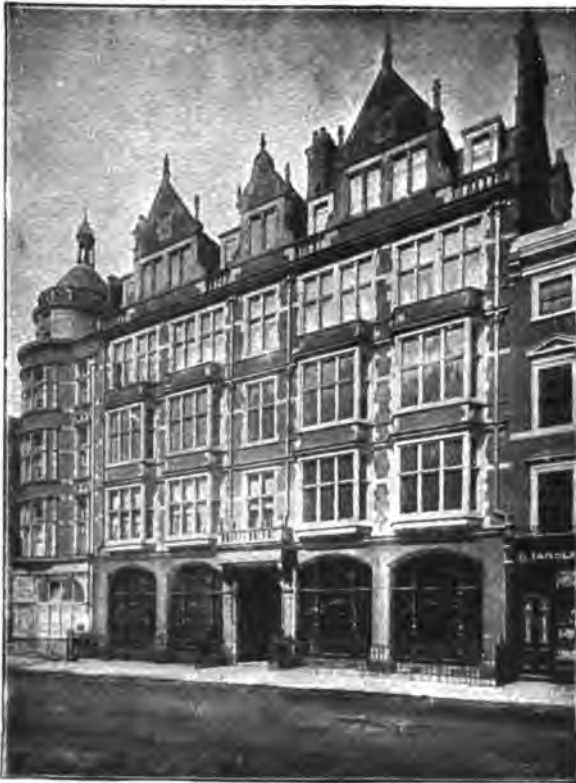
MESSRS. BRINSMEAD'S PREMISES IN WIGMORE STREET.
